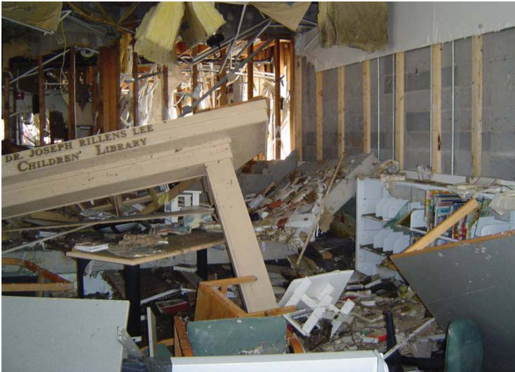
Waveland [MS] Public Library, Hurricane Katrina, September 2005
